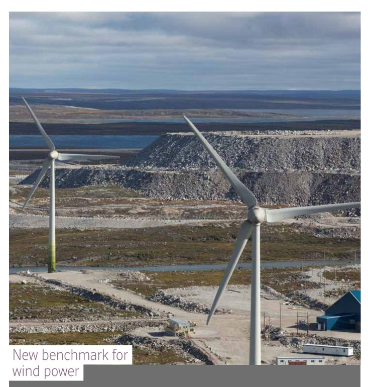
Supplying energy to the Diavik diamond mine in Canada's remote Northwest Territories is itself an energy-intensive process, as fuel has to be hauled over long distances. Diavik's solution has been to build the world's largest wind-diesel hybrid power facility. With four turbines featuring innovative de-icing technology that allows
