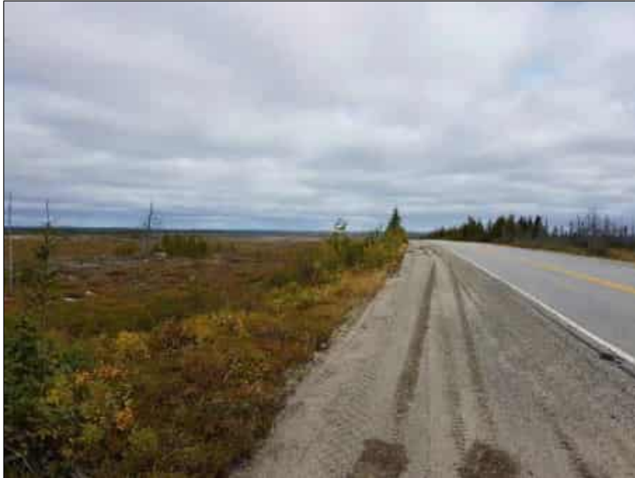
Photo 6-14 Road landscape unit
