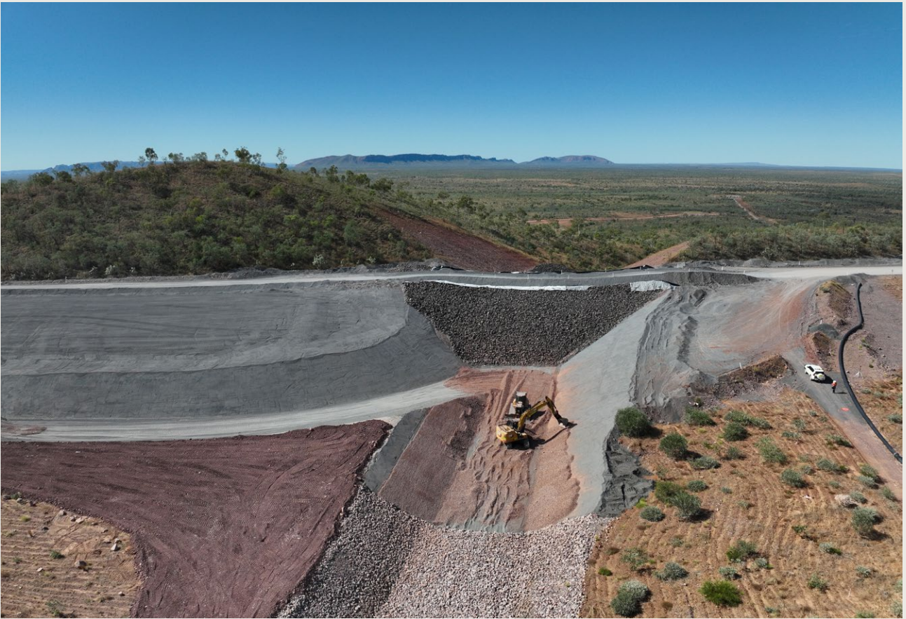
Above: Landforming works on the Telecom Ridge Spillway
