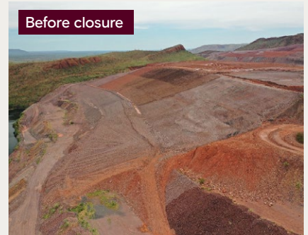
North Waste Rock Landform (2) North Central (NC)
