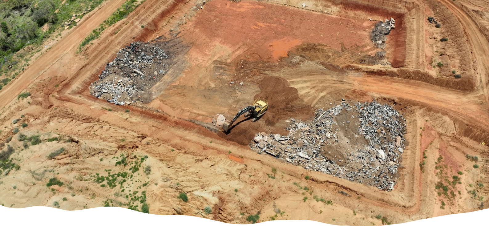
Above: Wandarrie landfill management. Below right: Asbestos removal at Argyle airport. Bottom of page: Transformer removal at the power station.
