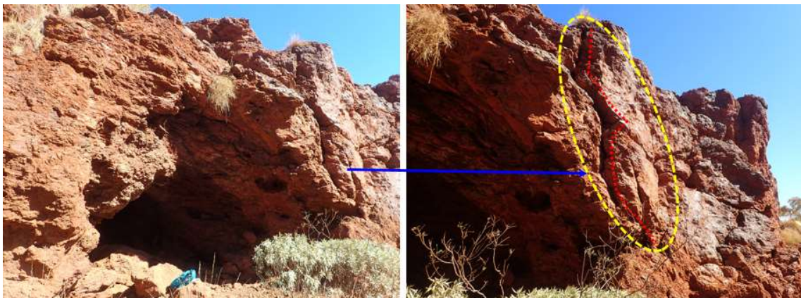
Figure 2 – Cave entrance and overview of the brow condition (left hand photo). Right hand photo highlights a large discontinuity and some defined blocks to the right of the entrance
