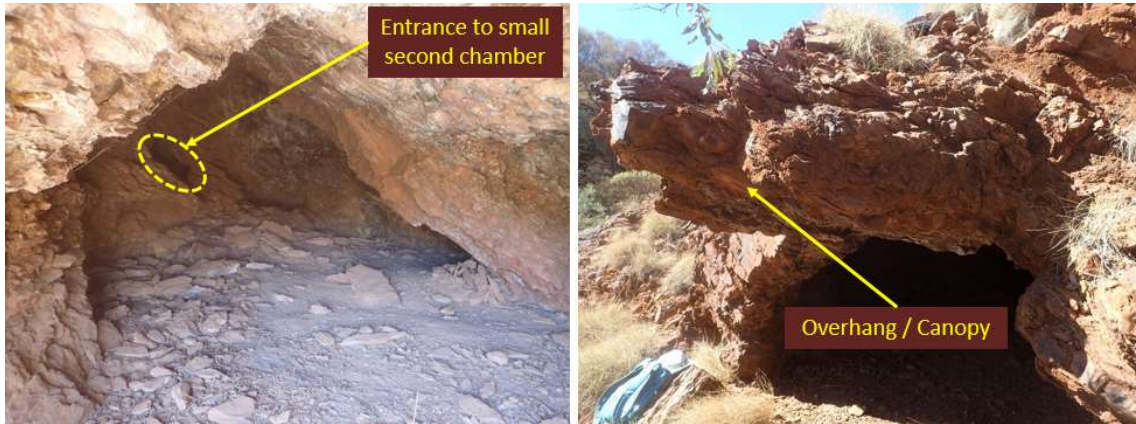
Figure 15 – View inside the main chamber and floor condition on the left. Total extent of the overhang / canopy in the photo on the right
