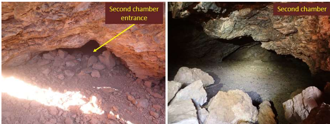
Figure 9 – Left: Entrance to second chamber and condition of first chamber floor. Right: view inside second chamber and condition of the floor (limited rockfalls)
