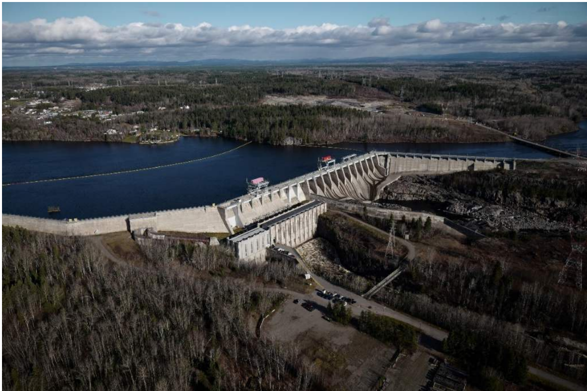
Image: Aerial view of the Chute-à-Caron hydro-electric power station. Saguenay, Quebec, Canada.
